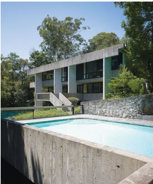
Figure 1 Seidler House, Killara (1966–1967), designed by Harry and Penelope Seidler in the mid-1960s. With large areas of unpainted board-formed concrete and dark framed windows, it resembles International Lodge. Photo by Brett Boardman (Source: Architecture.com.au)
